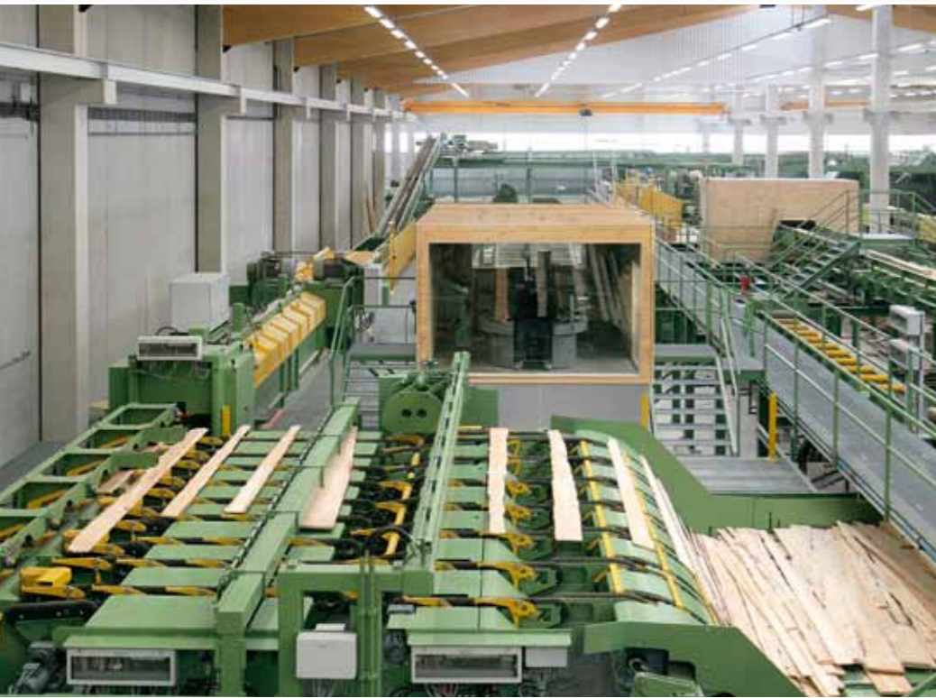
The whole OptiDrive Line is monitored from the operator control cabine protected from dust and noise
